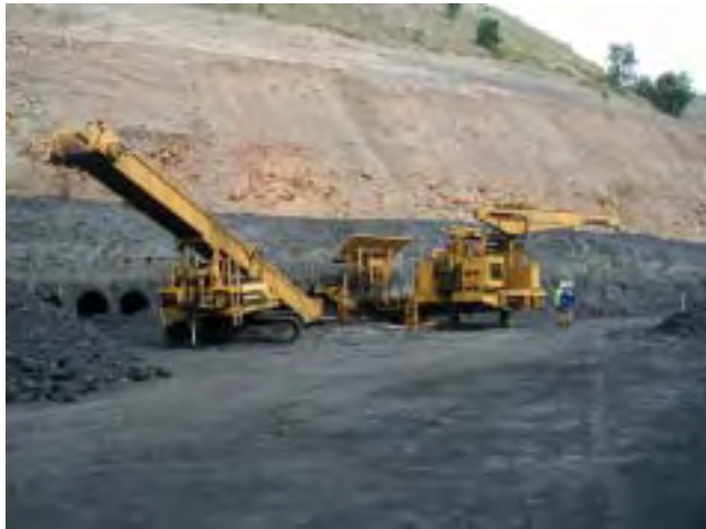
Highwall mining (steep incline auger mining system)
